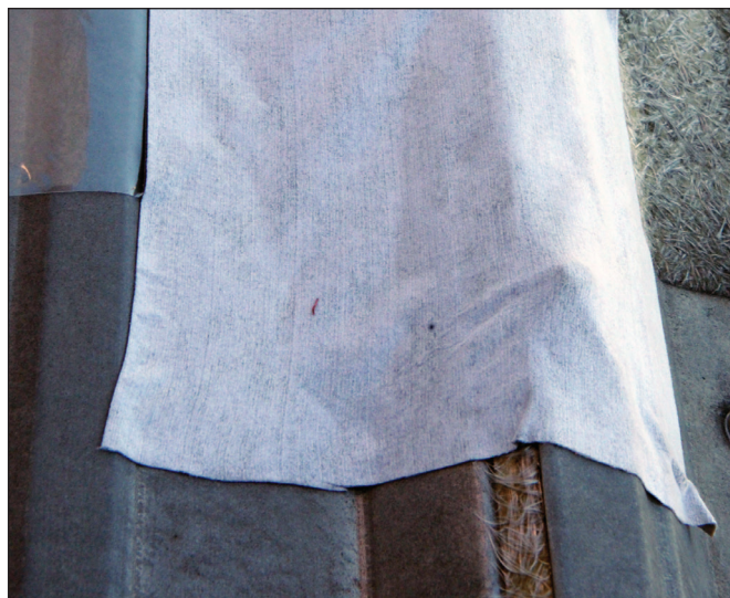
Seam Tape applied on metal roof seam
