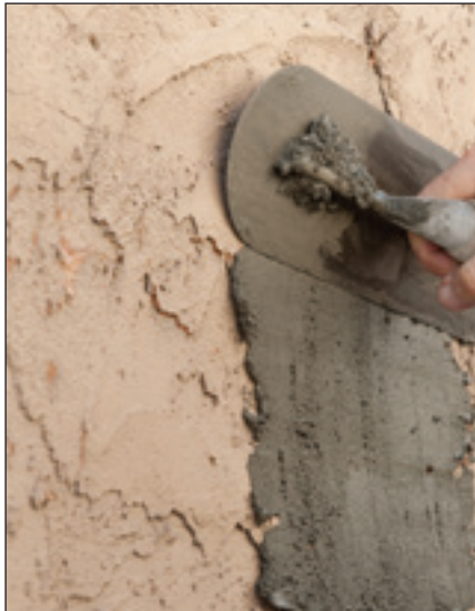
Sealopatch being applied to irregular surface
