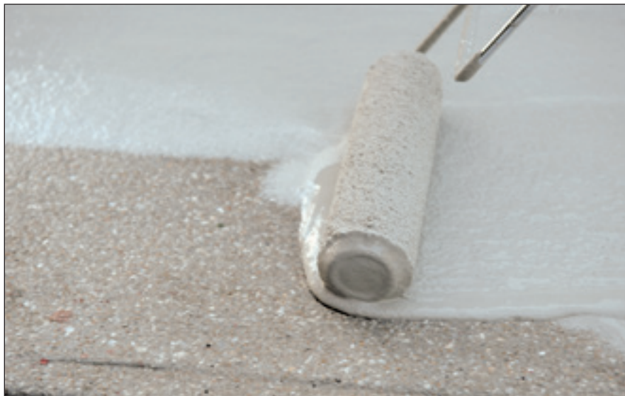
Sealoment Plus™ Being Applied Onto Concrete Walkway
