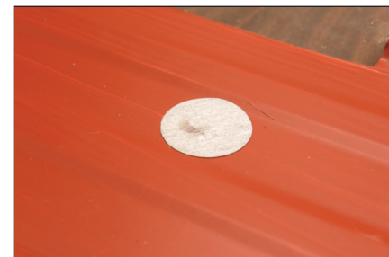
Sealocap installation over fasteners complete
