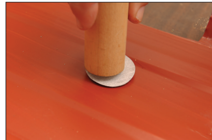
Use Sealocap Tool to adhere Sealocaps over fasteners
