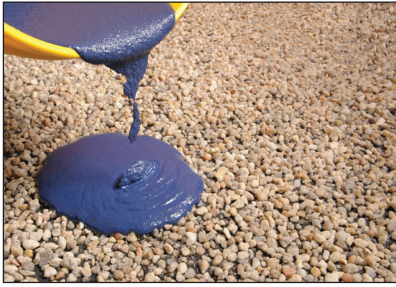
GRR Flood Coat being poured out of bucket
