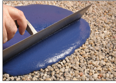
Spread GRR Flood Coat
