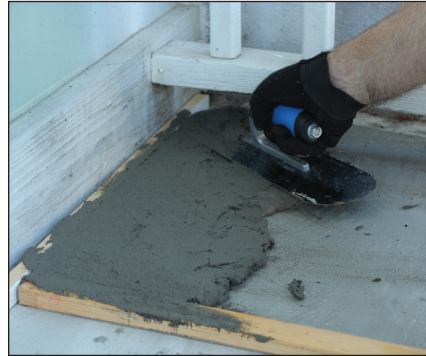
Flexobase being troweled onto deck
