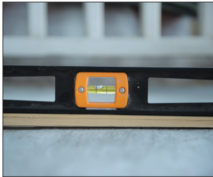
Note amount of slope on deck
