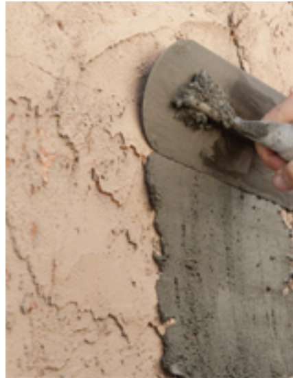
Sealopatch™ being applied to irregular surface
