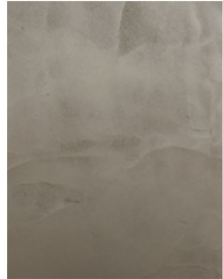
Surface after Sealopatch™ application
