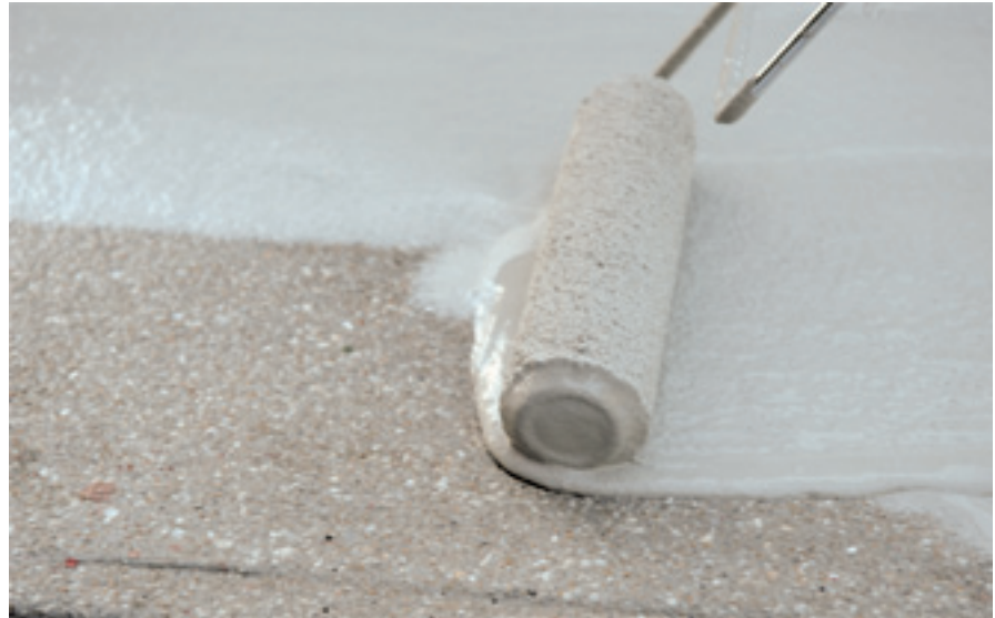
Sealoment Plus™ Being Applied Onto Concrete Walkway
