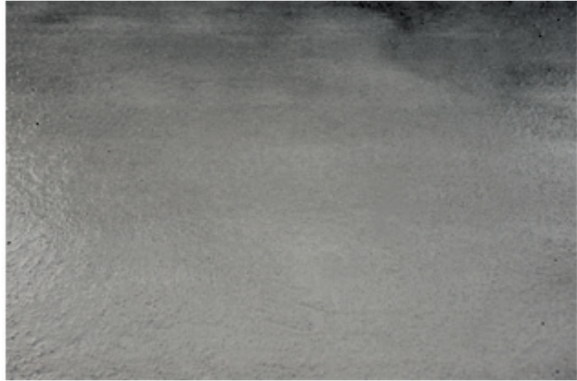
Sealoment Plus Application Complete
