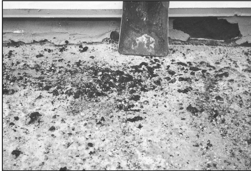
Gravel Roof Before
